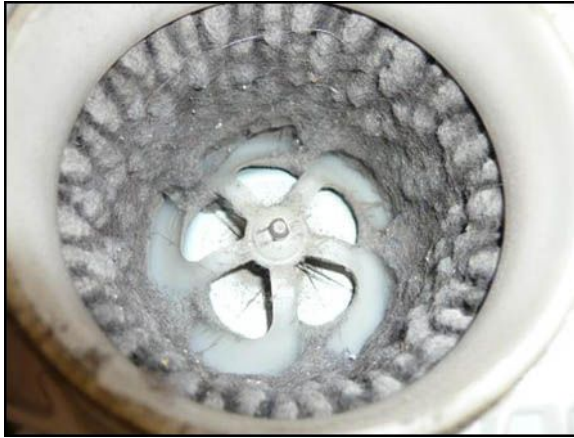
Figure 1. HV Battery Cooling Fan BEFORE Cleaning
